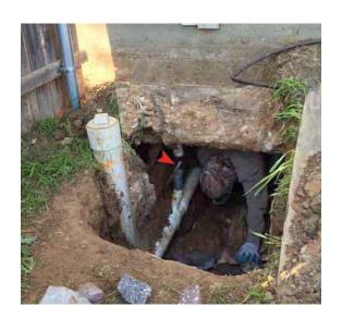
Prior to lifting, the utilities (gas, electric, etc) are exposed. This is to help prevent damaged during the lifting process. Utilities need the room and air space to move with the lift. Without this flexibility they will break. Notice where the arrow marks the ground surface.
