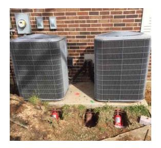
This is the A/C Pad after the home has been lifted. Notice how the A/C pad moved up with the lift.
