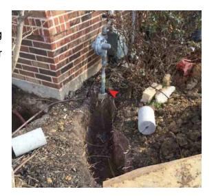
Notice where the arrow marks the ground surface after the house has been lifted. The utilities moved with the lift. There was no damage to the utilities during or after the foundation repair lift.
