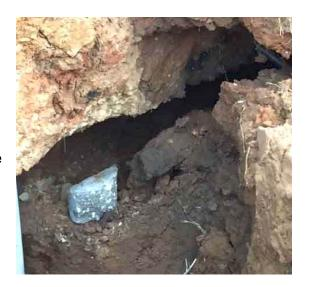
Hydraulic jacks go inside the tunnels. Placed under the foundation beams, they will lift the home to the correct level.
