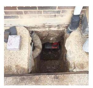
This is a foundation repair garage floor breakout. When completing a full-lift foundation repair, it is often necessary to break through the garage floor to reach the beam located under the garage. In this photo, two post tension cables have been exposed. The cables reinforce the foundation.
