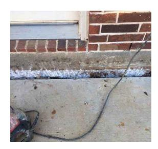
The house has been lifted a total of 12". Notice how the dirt along the back lifted up with the house; a full 12". Any plants, gate posts, or other objects next to the house would have been lifted, and would tilt away from the house. It is time for our crews to start the clean up. This is where it all starts coming together. In the foreground, we have lowered the dirt back to its original elevation. Any other objects that had been lifted out of position will also be put back to rights.
