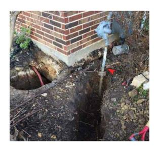
Remember the tunnels that were dug. They will now be used to access each beam under the home. Under slab tunnels are about 3 feet wide x 3 feet deep. It is just enough space to allow the technicians to maneuver under the home. Foundation repair pilings will be placed under each beam at 8-10 feet intervals.
