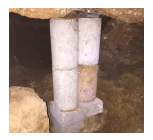
Notice the gaps that appear after the lift. Also notice the clean concrete exposed during the lift. Repairs to driveways and other flat work are done where needed.
