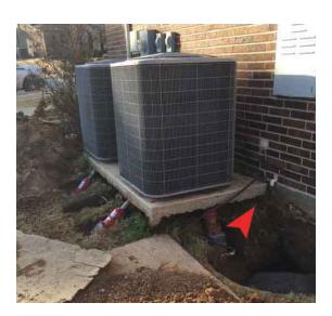
Once the foundation repair lift is completed, landscaping is put back in place and connections are covered back up with soil.
