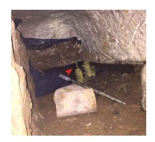
Support cylinders are then placed under the beams and shimmed to the proper height.
