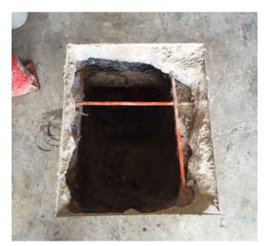
After the foundation repair lift, breakouts and driveway are repaired. The arrow is pointing to where concrete has been poured to cover the breakout.
