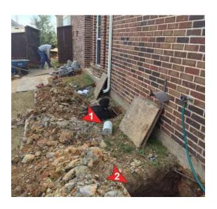
2. Tunnels are dug underneath the home. These run under the slab at intervals from one end of the home to the other. They are needed to gain access to all interior foundation beams.
