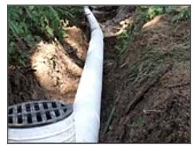
needed. Because pipes are smooth on the inside, they can move water away with slopes as little as one inch of drop for every ten feet.
